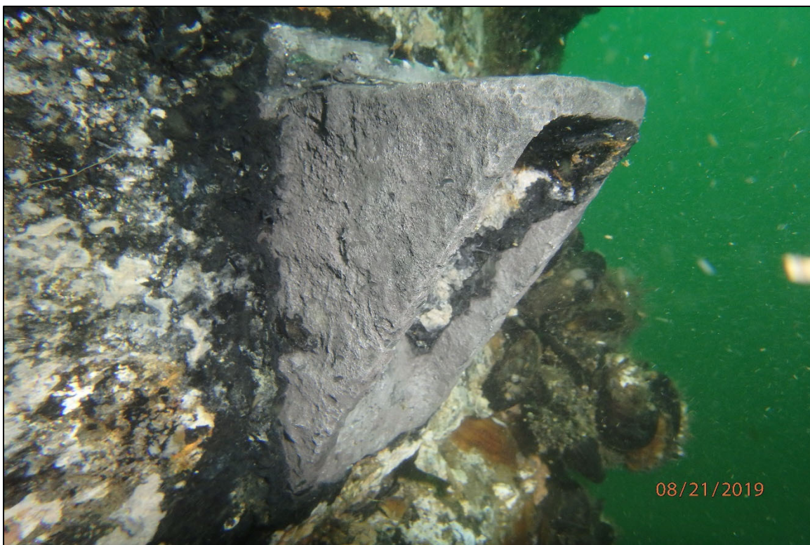
PHOTO 17. Typical Moderate Section Loss and Pitting on Diffuser Bracket, Taken at Diffuser E15 Southwest Anchor (Note Missing Bolt).
