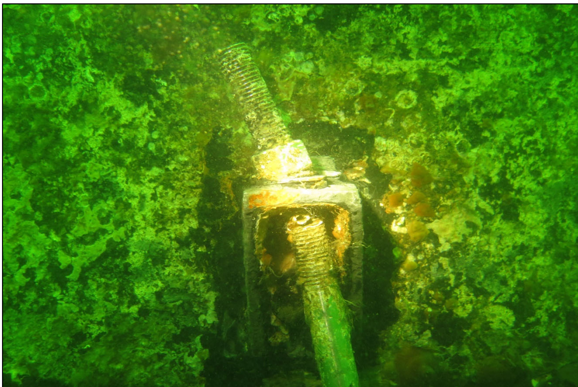
PHOTO 16. Stainless-Steel Anchor Bolt Bent with No Deterioration, Diffuser E3 Southeast Bolt at Top.
