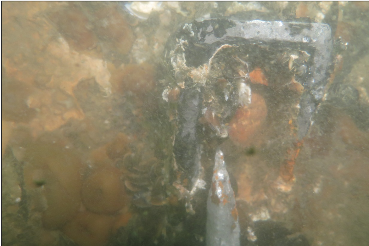
PHOTO 11. Typical severe corrosion with up to 100-percent section loss taken at Diffuser W13 southeast bolt at top bracket.
