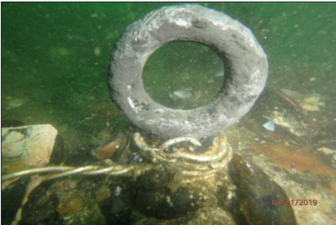
PHOTO 10. Typical Minor Section Loss on Padeye, Diffuser E15 South Padeye.
