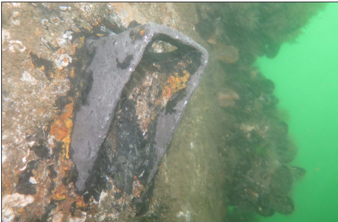
PHOTO 12. Typical Moderate Section Loss and Pitting up to 1/8 in. deep on the Diffuser Bracket, taken at Diffuser E27 southwest anchor.
