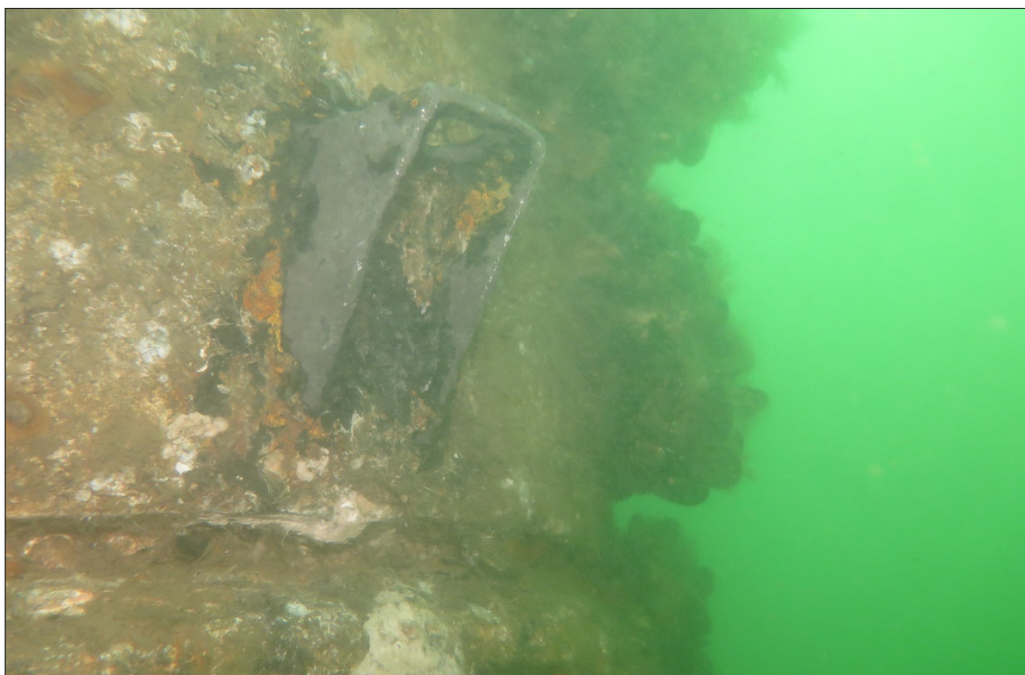
PHOTO 4. Diffuser cap/riser interface and steel hardware, missing the southwest anchor bolt, taken at Diffuser E2.
