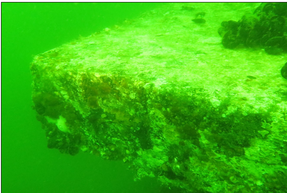
PHOTO 21. Typical Condition of Concrete and Rotation on Cleanout Chamber Cover, Taken at the Southeast Corner (Looking West).
