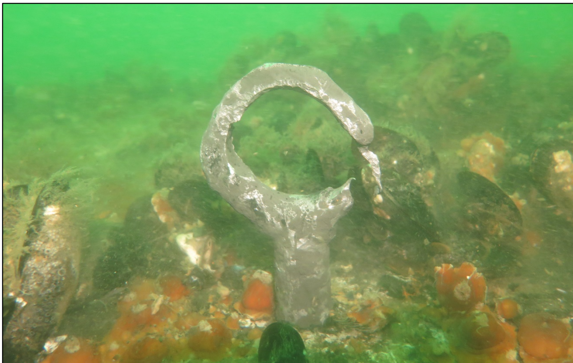
PHOTO 8. Typical severe section loss on padeye, Diffuser W13 south padeye.
