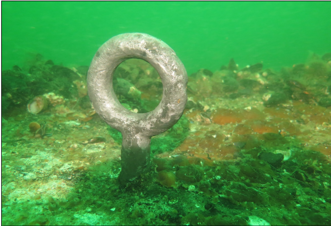
PHOTO 7. Typical minor section loss on padeye, Diffuser E29 south padeye.
