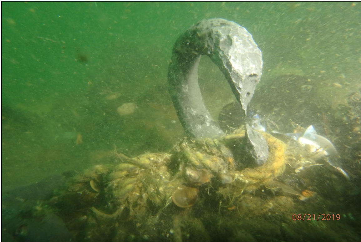
PHOTO 11. Typical Severe Section Loss on Padeye, Diffuser E15 North Padeye.
