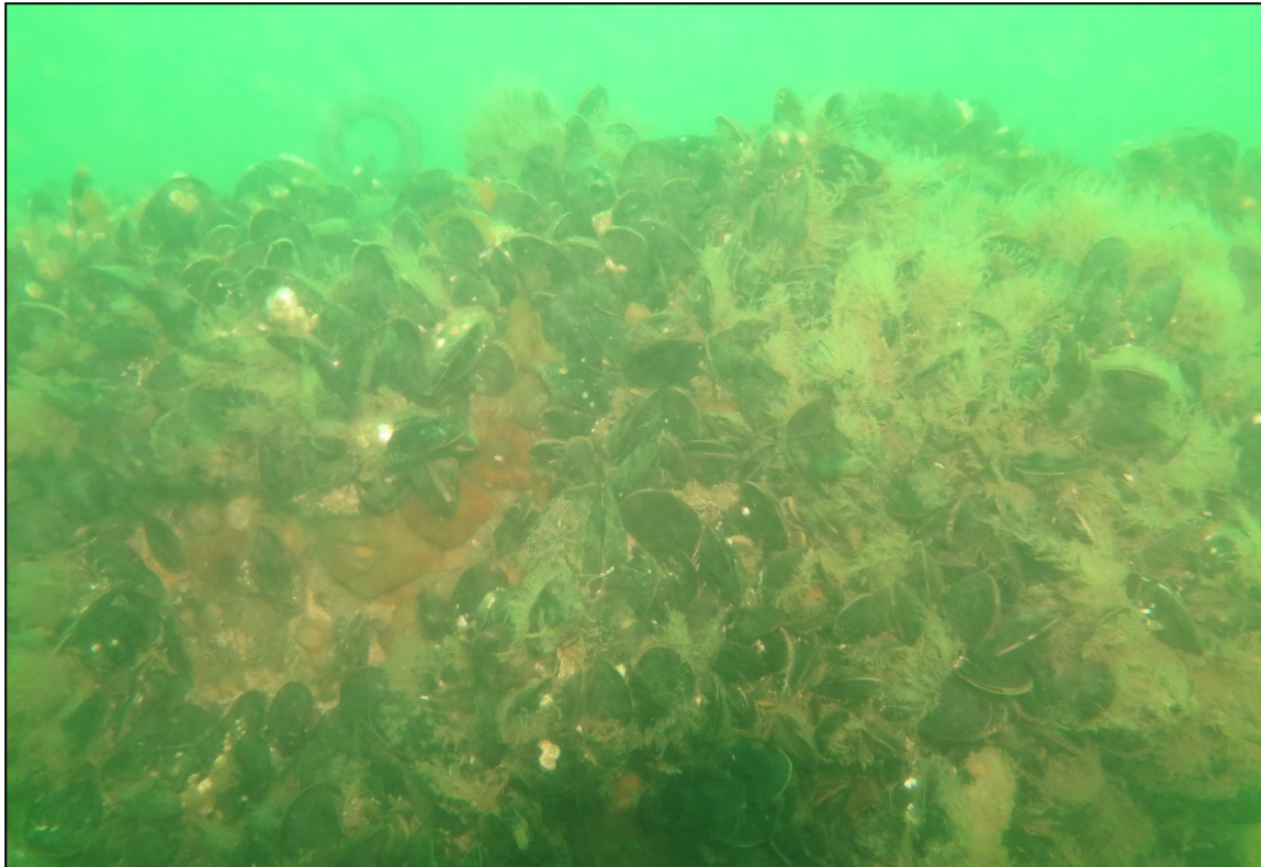
PHOTO 5. Typical outlet structure with marine growth, taken at Diffuser E29.
