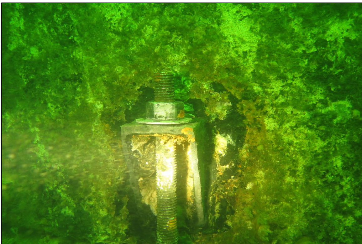
PHOTO 13. Typical Newer HDG Anchor Bolt, Taken at Diffuser E2 Southwest Bolt.
