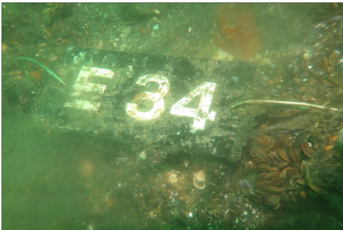
PHOTO 1. Typical I.D. tag on top of diffuser cap, taken at Diffuser E34.
