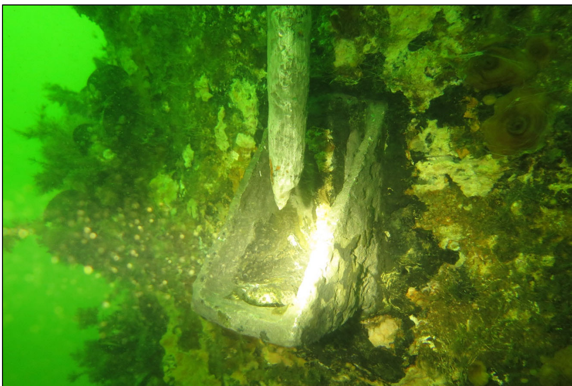
PHOTO 14. Typical Severe Corrosion with up to 100-Percent Section Loss, Diffuser E2 Northwest Bolt at Bottom Bracket.
