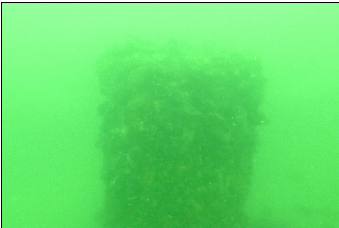
PHOTO 8. Typical Outlet Structure with Marine Growth, Taken at Diffuser E16.
