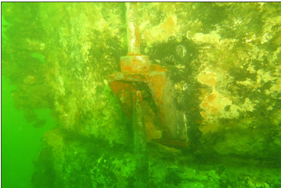
PHOTO 12. Typical Old Anchor Bolt, Taken at Diffuser E1 Northeast Bolt.
