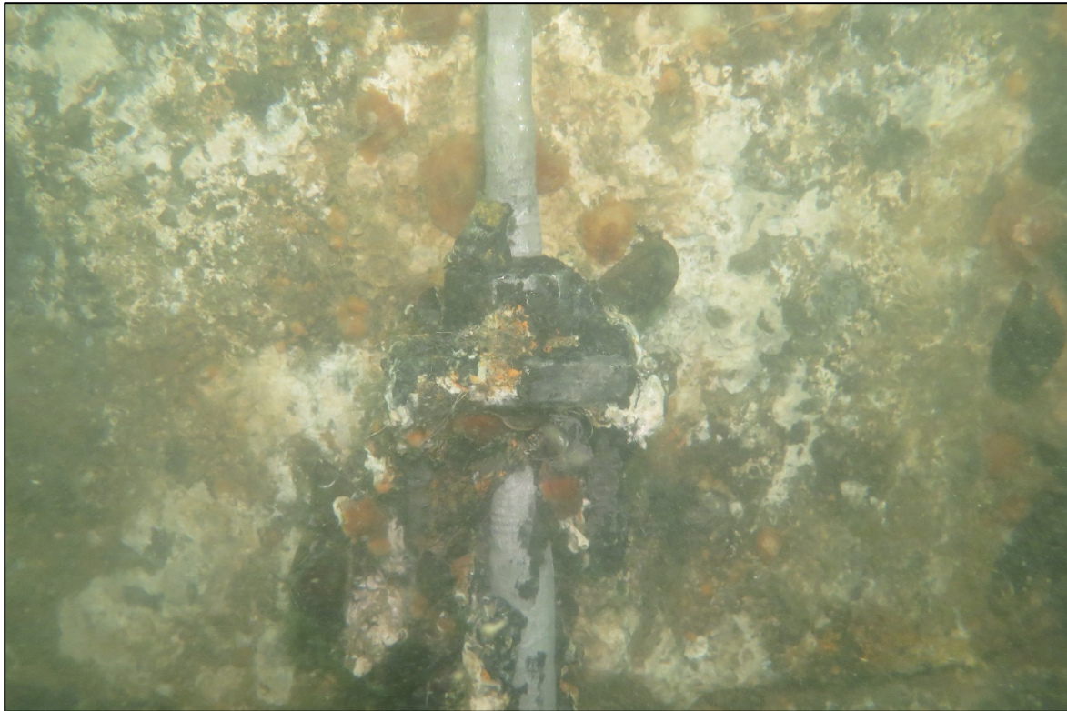
PHOTO 9. Typical moderate section loss on anchor bracket and anchor bolt, taken at Diffuser E29 southeast bolt.
