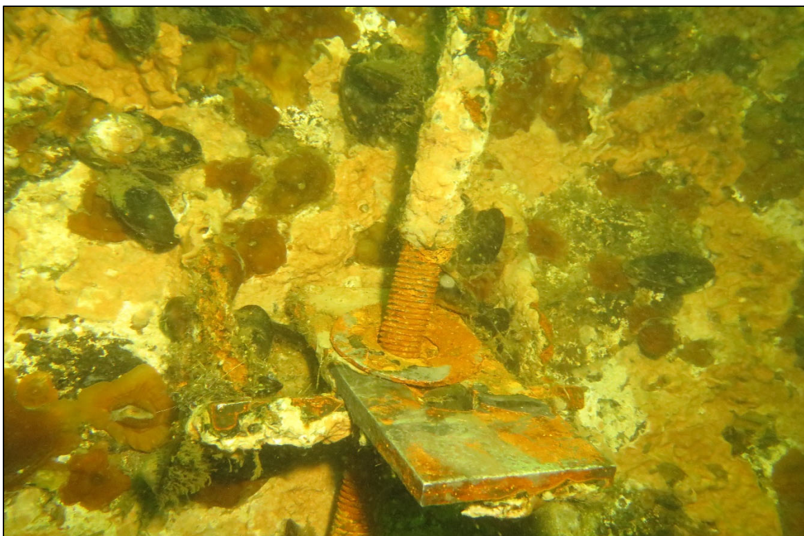
PHOTO 27. Typical Failed Anchor Bolt/Bracket W1 on the West Face of the Cleanout Chamber.
