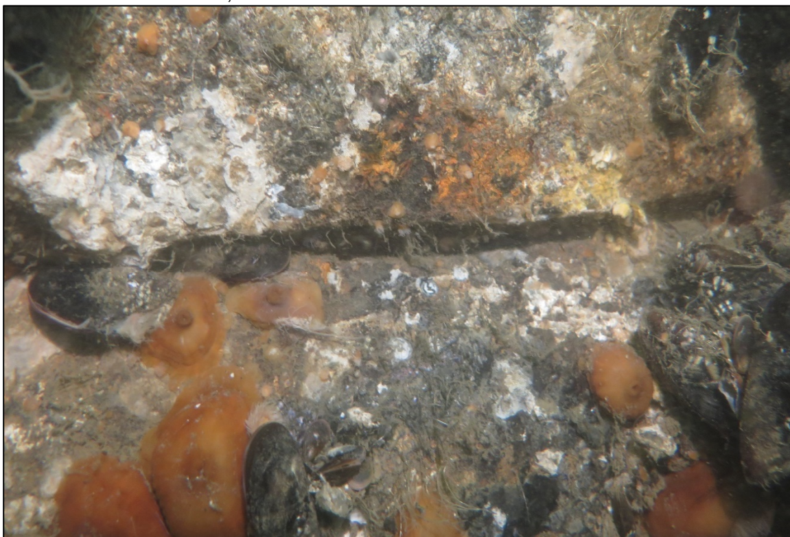
PHOTO 14. Typical condition of concrete on vertical face of cap on southeast side of Diffuser E29.
